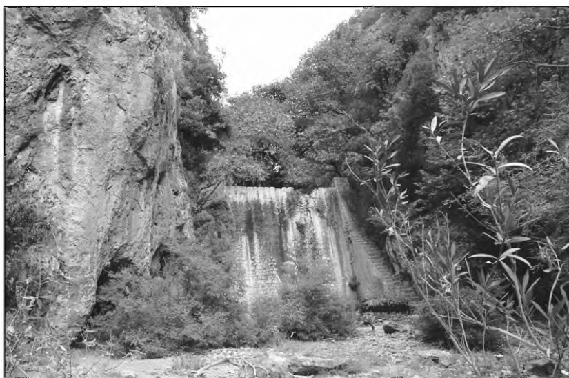
Figure 4. View of a dam in Nedon river; a major part of its basin was burned during the summer of 2007.
